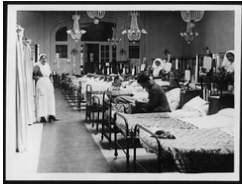
A ward in the South African Hospital
